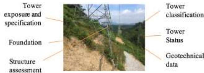
**Figure 2** Objects For Transmission Tower Assessment And Management Using Virtual Inspection
